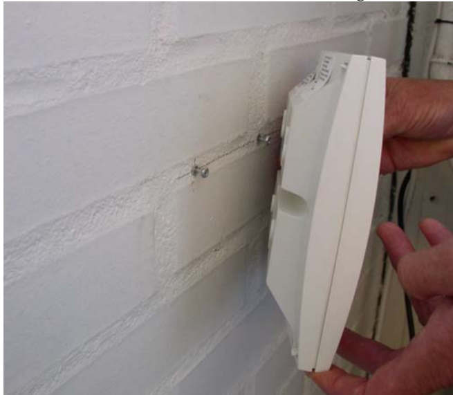
Figure 11 Wireless Server 600v3 Wall Mounting
